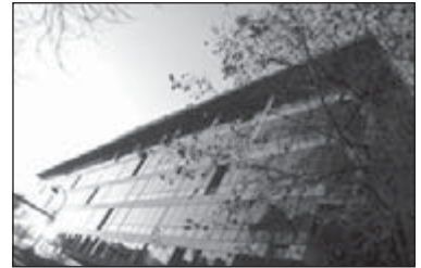
Work advances on restoration of the main office building.
